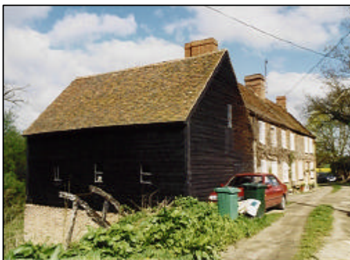
Note the remaining fragment of a quarter of the water wheel framework in the pit at the side of the mill
