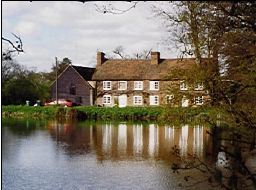
Flanchford Mill and Cottages and Flanchford Mill, 1999
